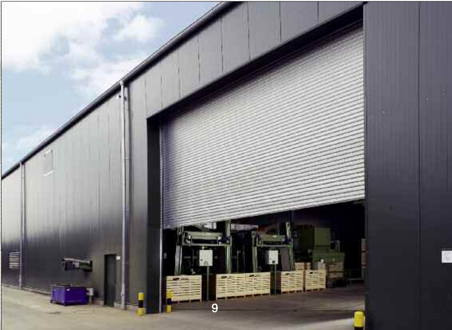
Door opening in an industrial premises.
