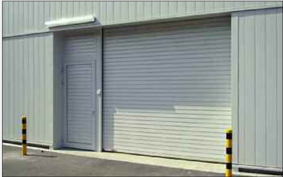
Roller door with fixed side door.
